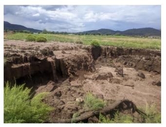
Servere Erosion Damage - Copeland Detention Facility Page 137 of 222
