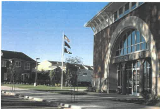
Fairview Village City Hall and nearby housing.
